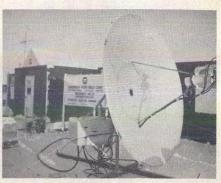
1. Small dish earth stations in Alaska can be installed without disturbing the tundra. Less than 5 W of power is required per carrier for satisfactory uplink C/kT with a 15 ft dish. The channel capacity for thin route service to small stations is between 220 and 460 simplex channels per 5W transponder, depending on location.
