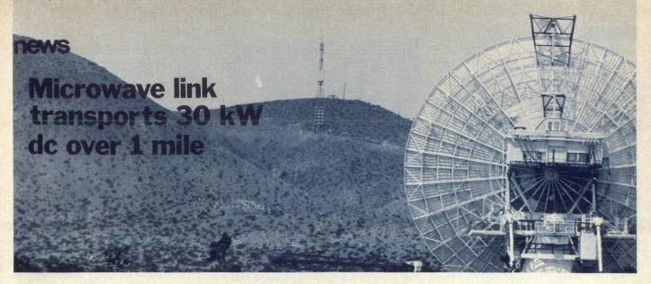
This 85-ft dish at Goldstone transmits 320 kW at 2.388 GHz to the rectenna array mounted on the tower in the distance, over a mile away. Intercepted rf to dc efficiency is over 80%.
