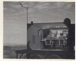
5. Aquila program will use two operators located in a portable shelter to control the vehicle. The RPVs progress is portayed automatically on an X-Y plotter that has a map behind it to help the operators follow the waypoint navigation.
