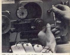
UTI checks the cores of all Micro-Coax cables to assure the concentricity of the center conductor within the dielectric. Consistent characteristic impedance throughout the entire cable length is just one of the advan-
