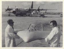
11. Subsonic delta wing mini-RPV developed by Teledyne-Ryan for Navy's STAR's program weighs 120 lbs to 140 lbs depending on payload. It's wings measure 7 1/2 ft. from tip to tip. It's constructed of plastic foam for minimal radar cross section and ruggedness. It's designed to fly at altitudes from 100 ft to 10,000 ft carrying TV/laser designator payload weighing up to 50 lbs.
