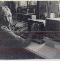
3. Instrumentation for measuring the power transmitted and received includes this Interdata computer. The display presents input rf power, output dc power, efficiency, voltage and temperature at the rectenna ele-ments. Dc readings are separately calibrated to 0.5%.
